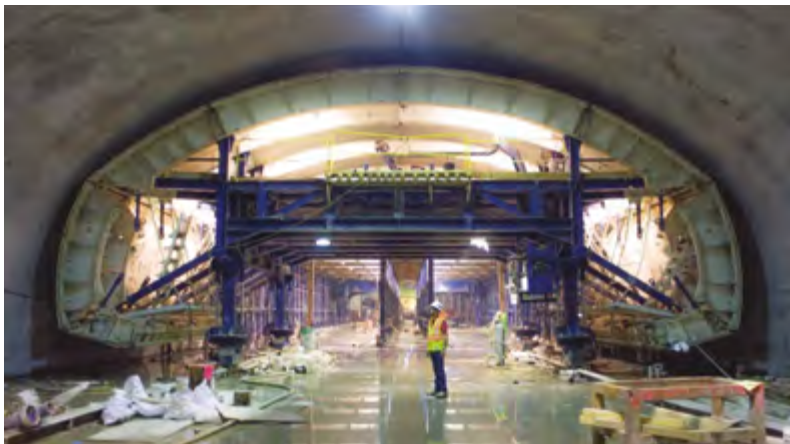
Under construction of the 2nd Avenue subway line, New-York, 2013. MTA Capital Construction/Rehema Trimiew/Wikimedia, CC BY-SA
